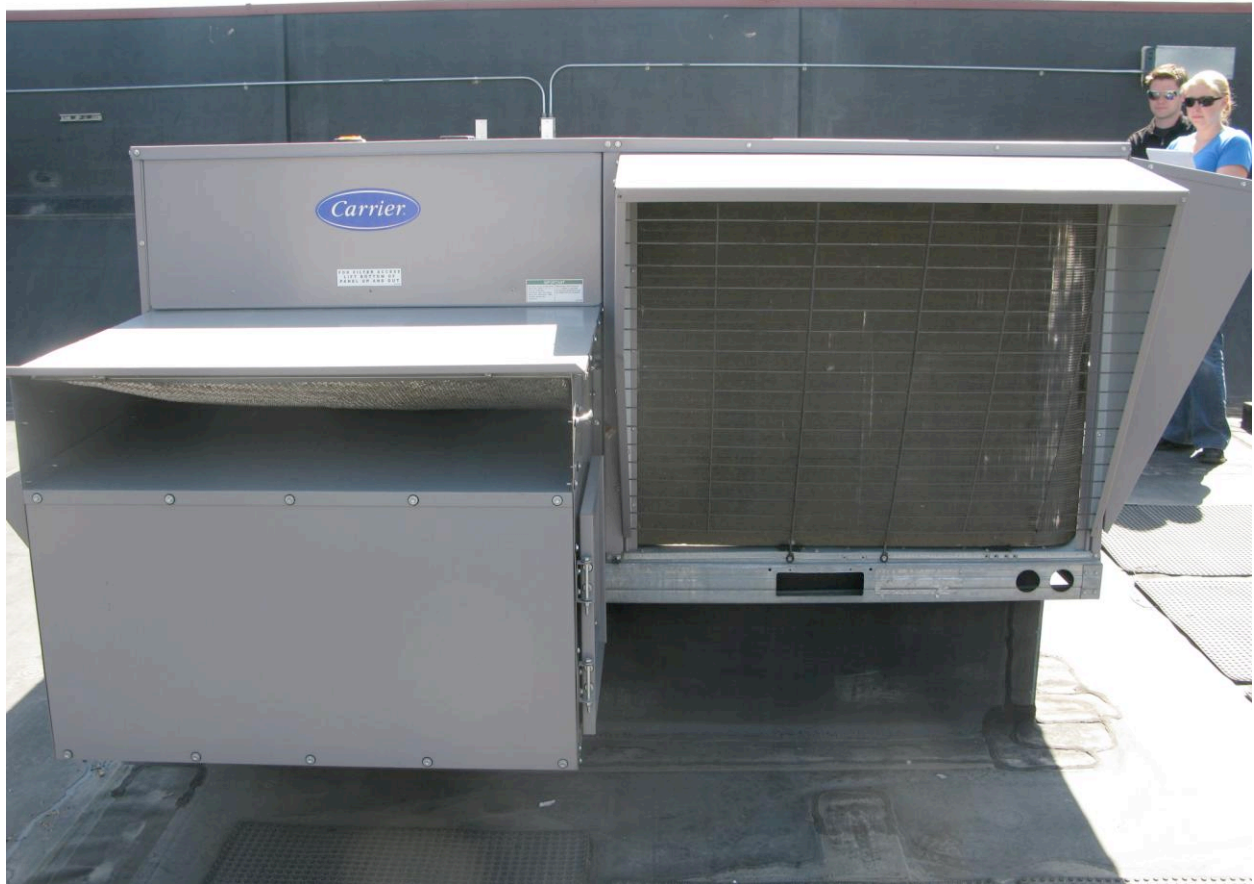
Central Air 3 Phase A/C Unit – Carrier Model #48TMD009 – 501NB 208 Volts 20 Amp
