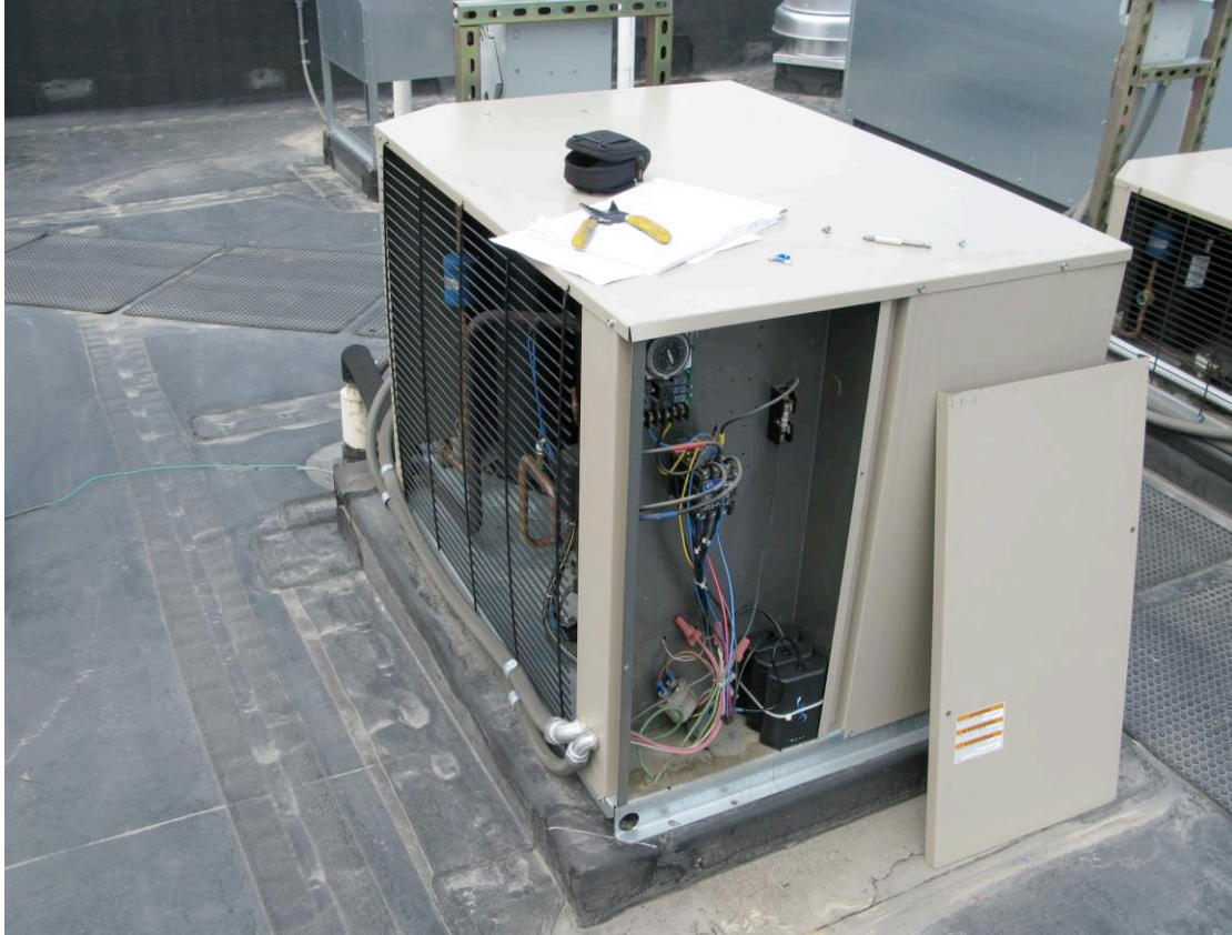
Heatcraft Refrigeration Products Beverage Walk In Cooler Model #MOH040D73CFT (3 Phase) – 208 Volts
