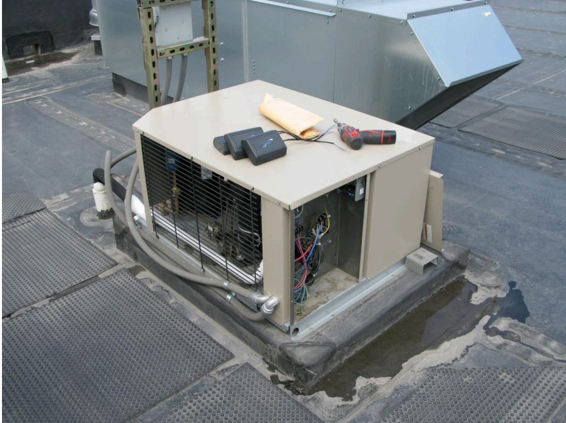
Heatcraft Refrigeration Products Beverage Walk In Cooler Model # MOZ035L63GF (3 Phase) – 208 Volts
