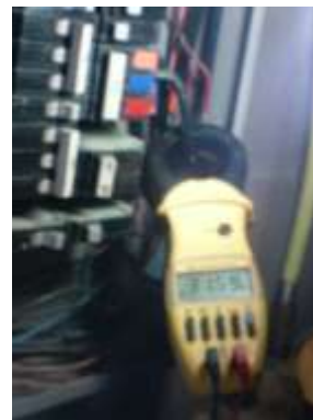
Side Wash Cycle 31.23 before & 25.57 after, 5.66 Amp reduction
