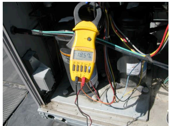
Reading after install (18.57)
